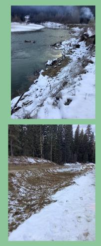
Example of a road upgrade project that was moved from spring 2022 to fall 2021. Staff was concerned the existing road may affect the adjacent stream during spring run-off. The photo above shows the state of the stream bank while the other image shows how the existing road will become an armored embankment with the new road well positioned away from the stream bank.
